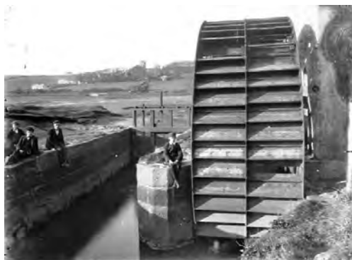
old sluice gate
