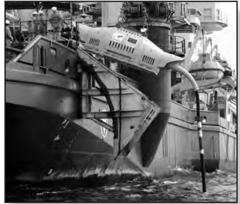
Above: Wave Hub being overboarded
